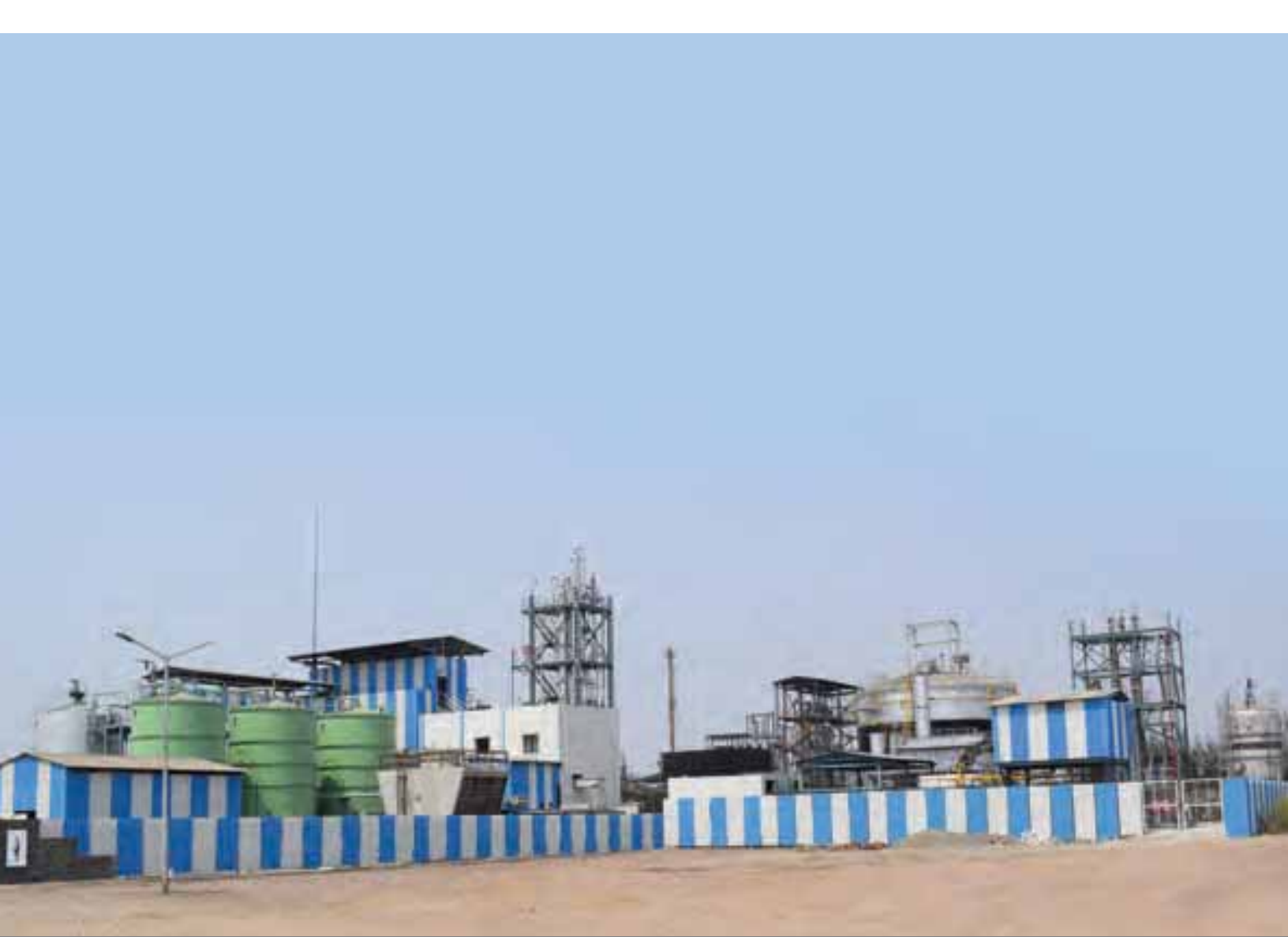
Praj's 2 nd Generation Biorefinery Demo Plant
