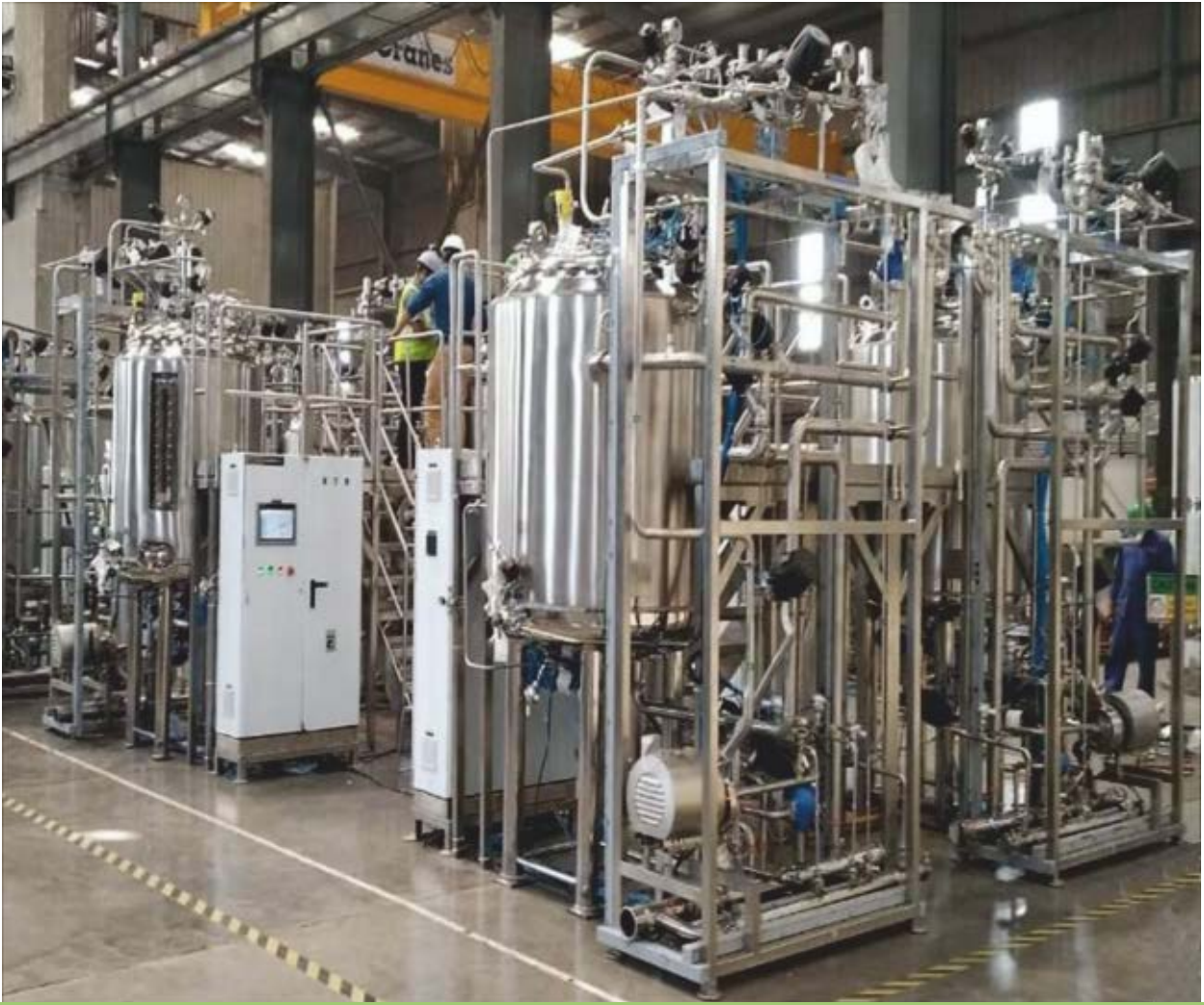
Sterile Water System and Process Skids for Vaccine plant manufactured at Praj HiPurity System's Wada (Thane) facility. The systems has been designed as per USFDA and WHO norms.
