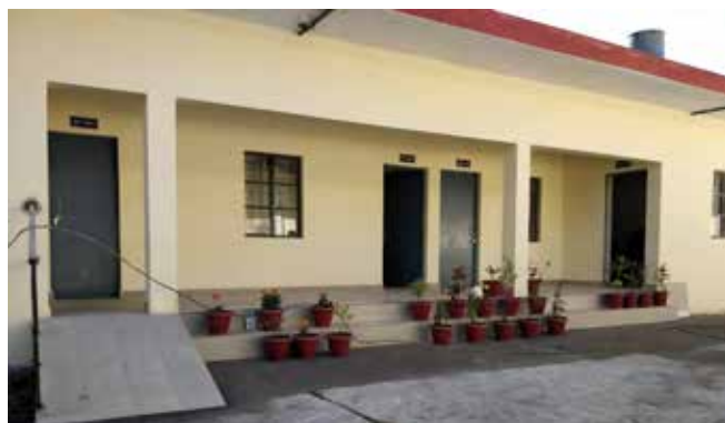
Godowns constructed by FCI under Central Sector Scheme at Tanda Kholi, Kangra, Himachal Pradesh
