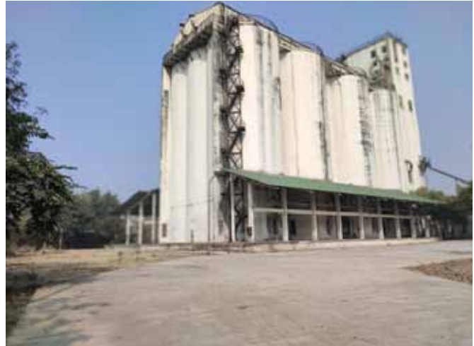
A view of Cement Silo
