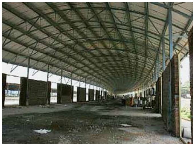
RWC, Jogeshwari, Mumbai, under construction
