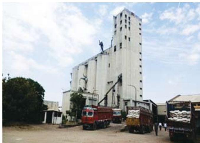
SILOS storage facility of FCI
