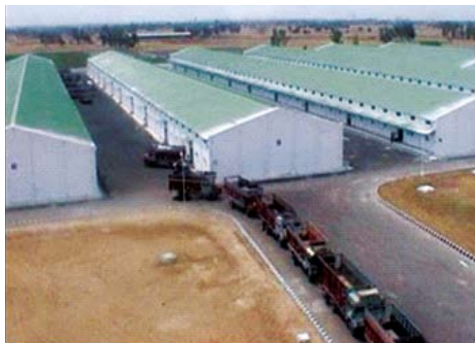
Construction of Storage godowns under PEG scheme
