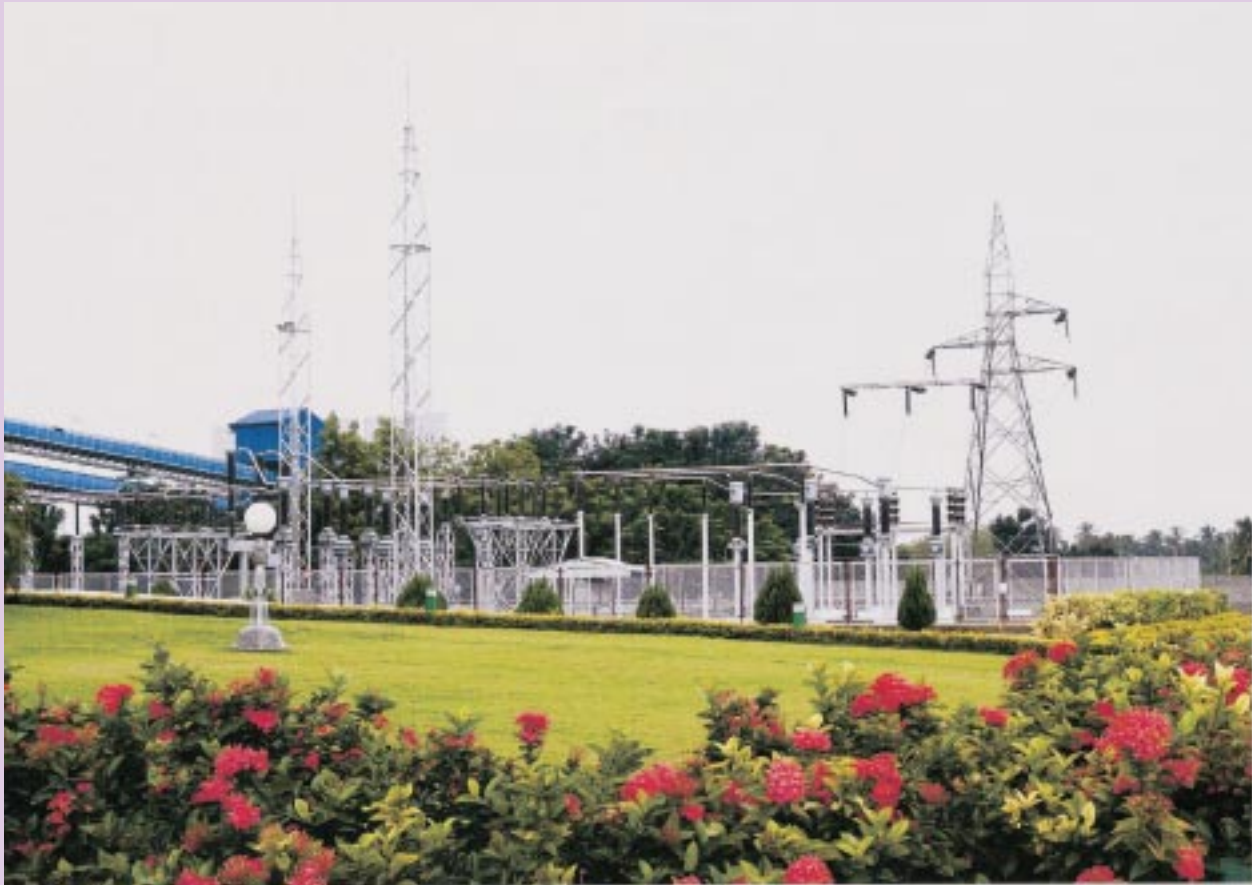
Sugar Mill Cogeneration Power Plant - Interfacing with Grid
