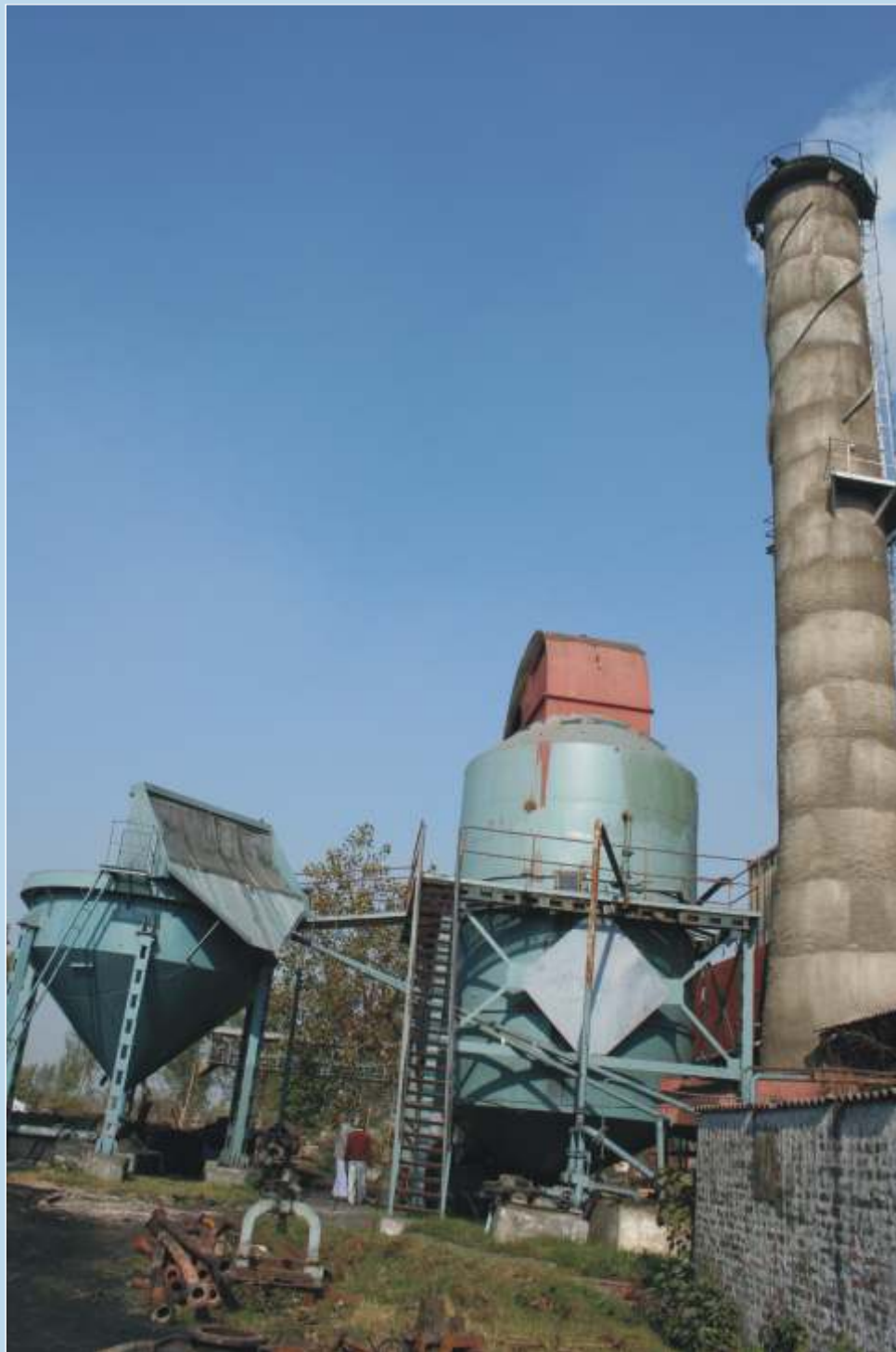
Air Pollution Control Unit of a Sugar Factory
