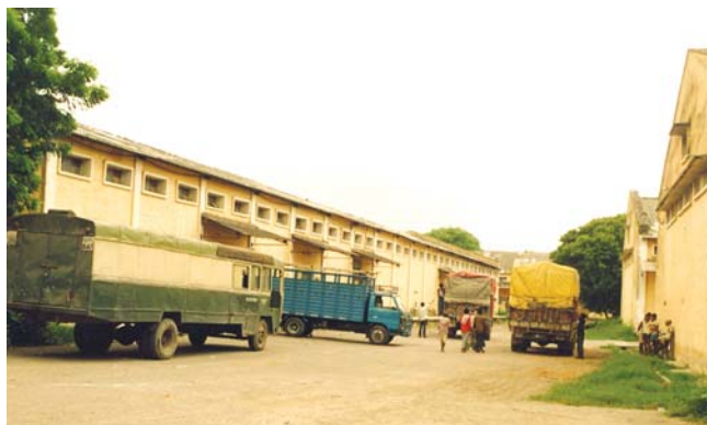
A view of foodgrain warehouse
