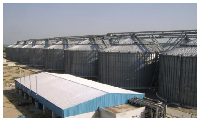
Silo storage facility for foodgrains
