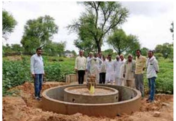
Community Recharge Structure serve rain water harvesting. These structure constructed to increase the ground water table.
