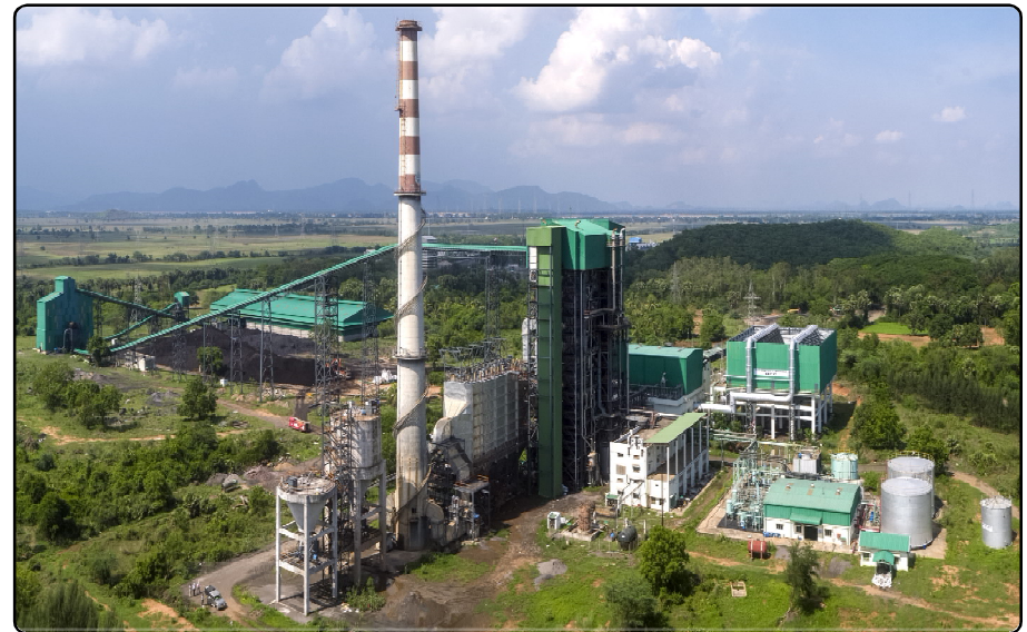
Thermal Power Plant at Saggonda
