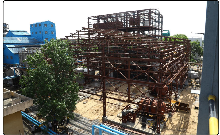
Salicylic Acid Capacity Expansion Project (under Construction) at Tanuku
