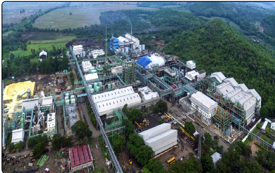
A Bird's Eye view of Chemical Complex at Saggonda
