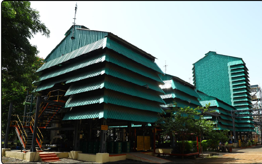
Rocket Propellant (HTPB) Production Plant at Tanuku
